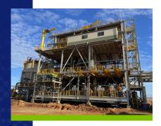
The Atlas Mine forms part of the Atlas-Campaspe Project, which began extractive mining in 2022 with a project mine life of 10 years. A dry mining technique is used to extract ilmenite, rutile, leucoxene and zircon from ancient coastal deposits. The ore is initially concentrated at site before the heavy mineral concentrate is trucked to the Ivanhoe rail siding, where it is then transported via train to the Mineral Separation Plant at Broken Hill.
