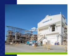
The plant produces approximately 140 kMT of titanium dioxide ( ${\rm TiO_2}$ ) annually, through the chloride process, which uses chlorine to react with titanium-bearing ores. The  ${\rm TiO_2}$  based pigment is then surface treated, dried, and milled to a uniform fine white powder. The finished product is then packaged and distributed to our customers by rail or sea from warehouse facilities at the Port of Fremantle.
